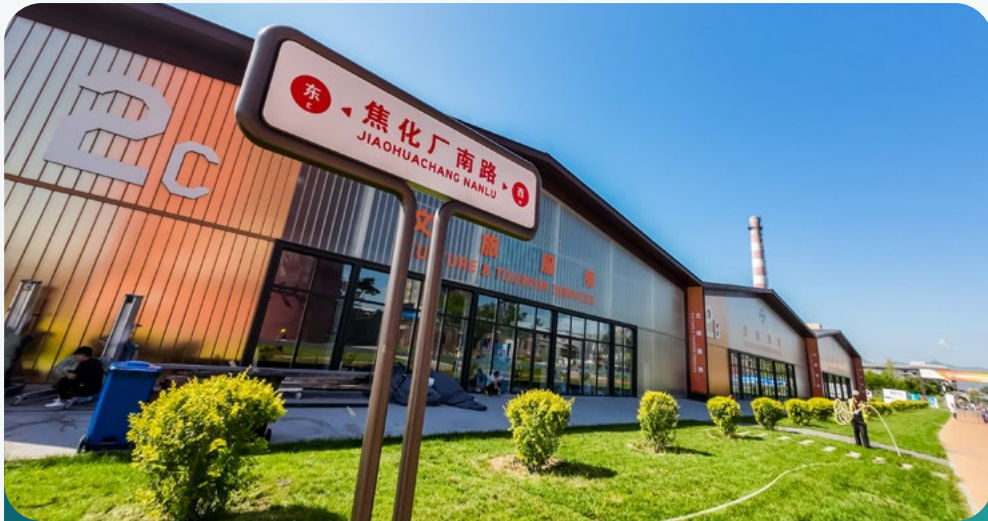
The views of the Shougang Park
