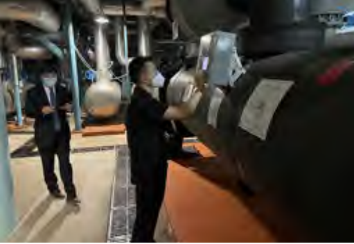
Carried out safety inspection
